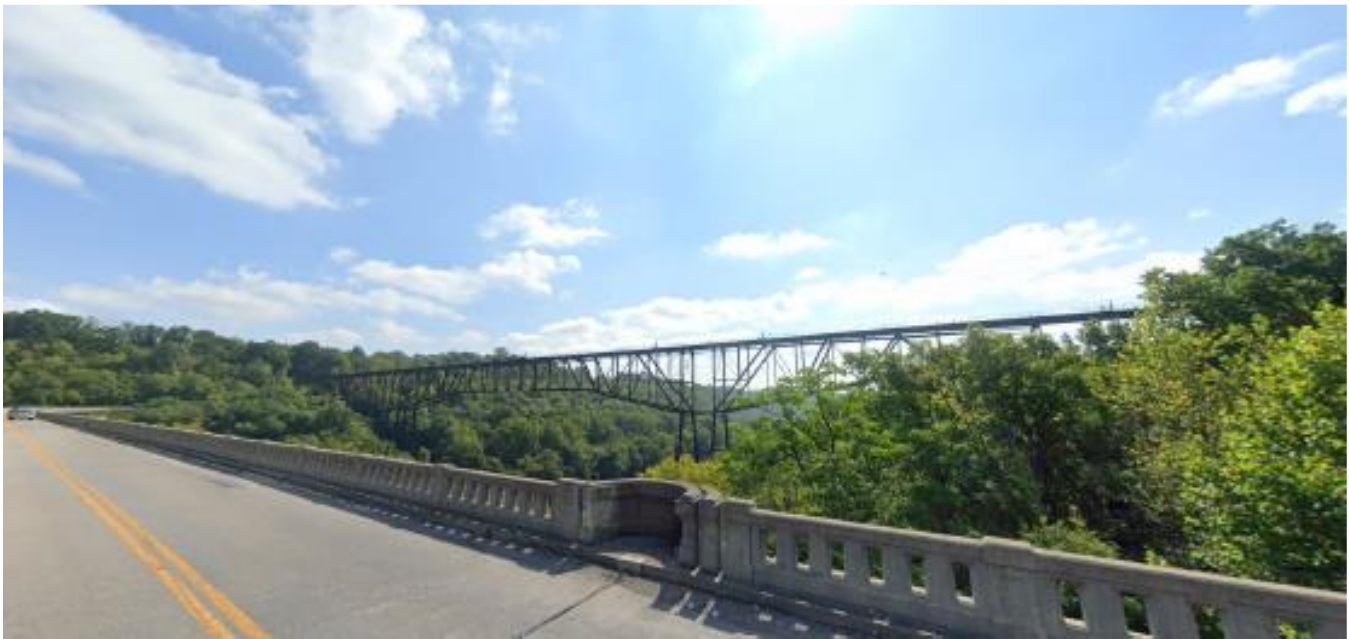
Figure 23: Youngs High Bridge
