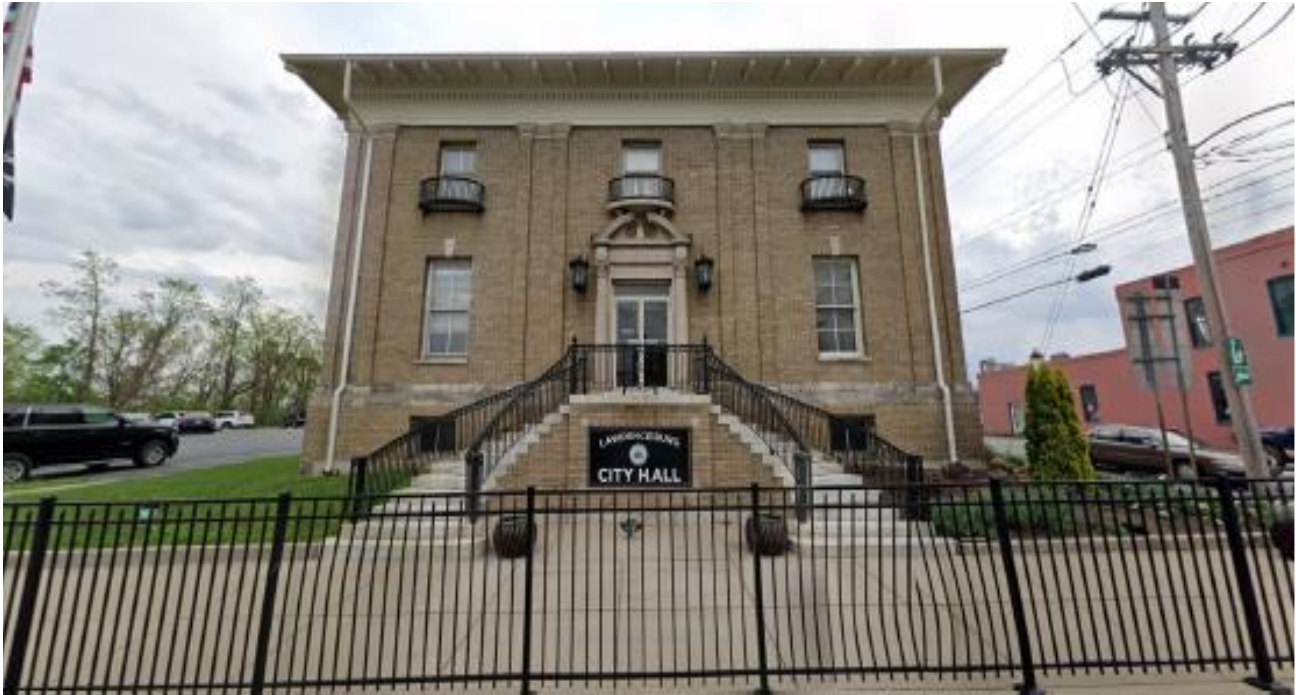
Figure 18: Lawrenceburg City Hall
